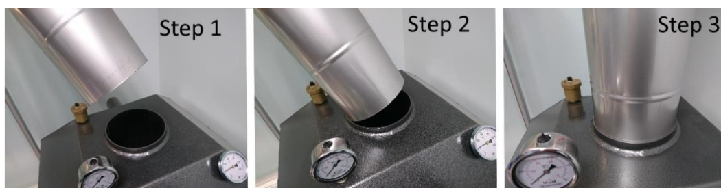
Image 4. Chimney installation
