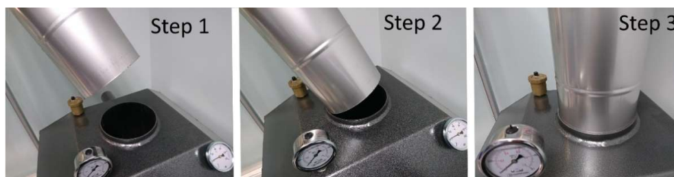
Image 4. Chimney installation
