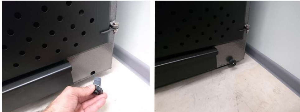
Image 5. Location of the drain plug
